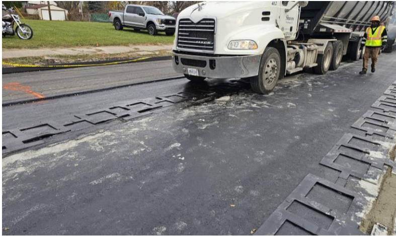
14 th St. Dynamic Charging Installation
